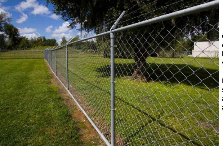
Galvanized chain link fencing is the most common type of chain link fence that you would normally see in a backyard. This is the silver looking chain link fence that you see many places.
